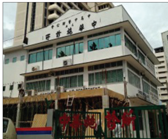
Figure 6: Original Chinese Medical Aid Department (中华施诊所) The building was burnt to ash in a fire incident in 2017)
